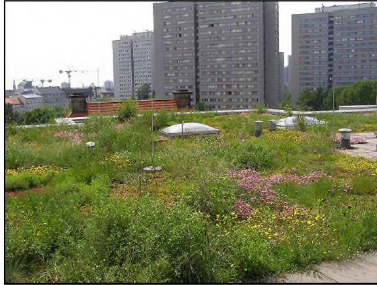
INTENSIVE GREEN ROOF PLANTED WITH PERENNIALS
